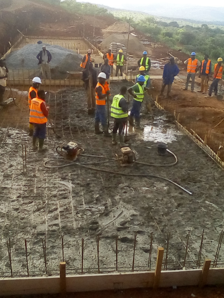
Construction de la station.
